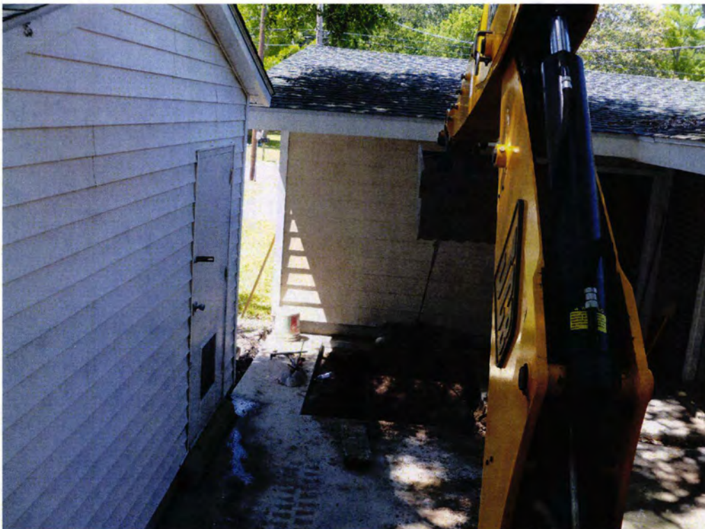
Picture 2: UST 329Ash extraction in progress.
