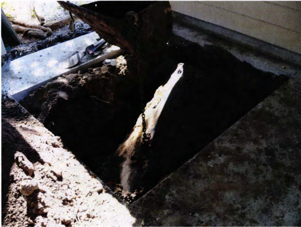
Picture 3: UST 329Ash extraction in progress.
